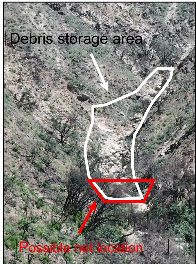
Figure 6. Choke-point in channel with upslope storage.
