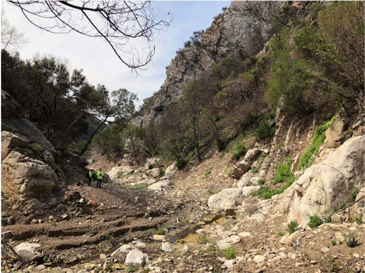
Site SY-7 Photo by Kane Geotech (2018.05.29)
