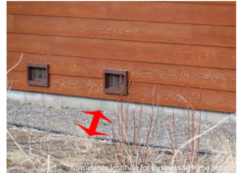
A noncombustible zone around a home in the Lake Tahoe Basin. In this case, requirements related to water runoff and protection from wildfire align.
