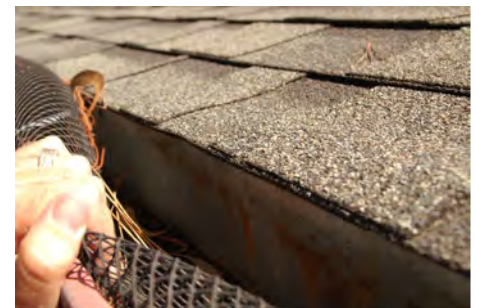
Gutter with integrated drip edge. Source: firecenter.berkeley.edu/bwmg/gutters.html
