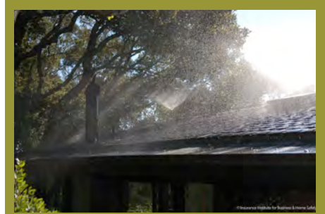
Photo 1. Roof mounted sprinkler.
